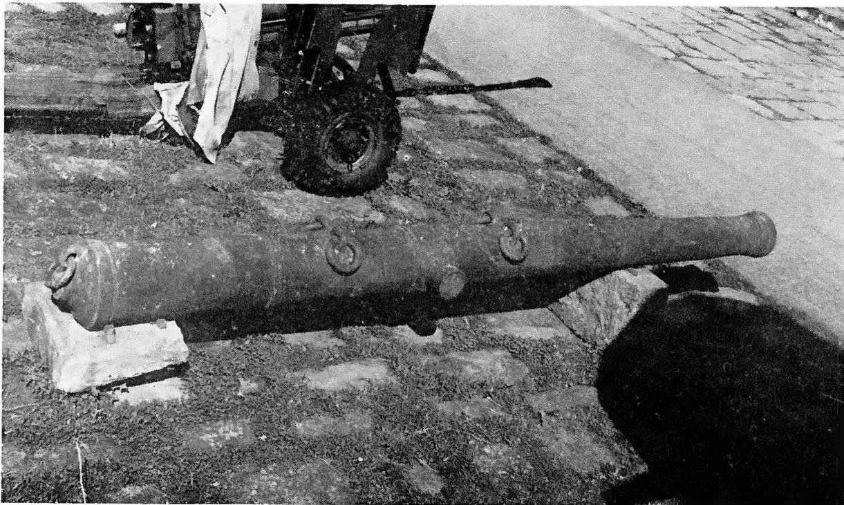
2 — PORTUGUESE BRONZE CULVERIN. Length 3,62 m.  $\varnothing$  11,5 cm. The Arms of the kingdom of Portugal and a sphere, in relief, between the muzzle and the trunnions. Four rings on the barrel and a ring on the breech.
